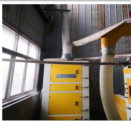
喷砂废气除尘滤筒
